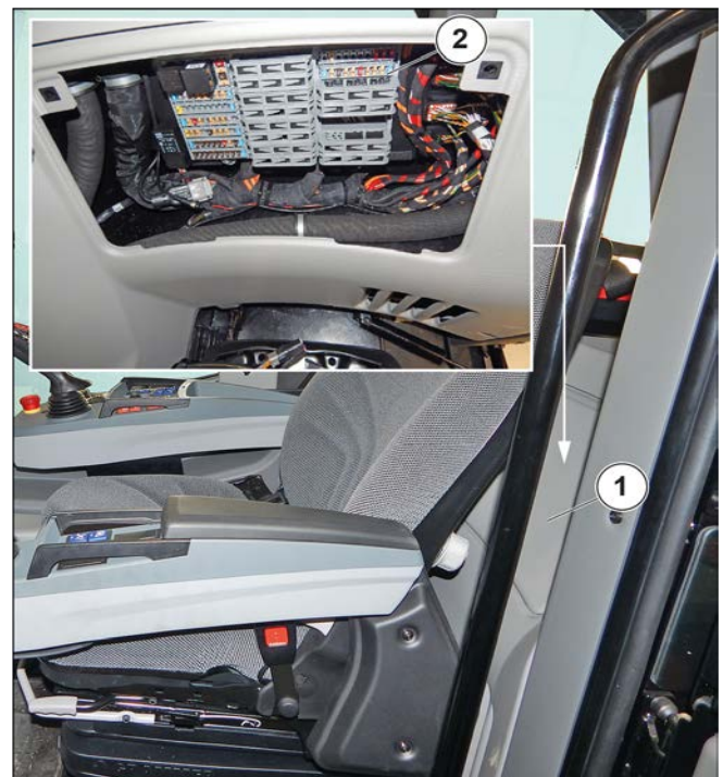
Figure 214: Fuse and relay in cab
