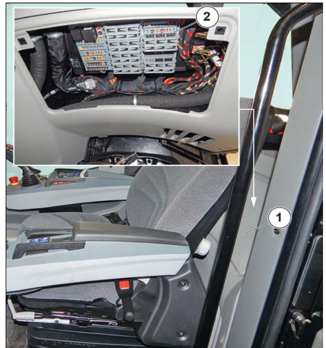
Figure 214: Fuse and relay in cab
